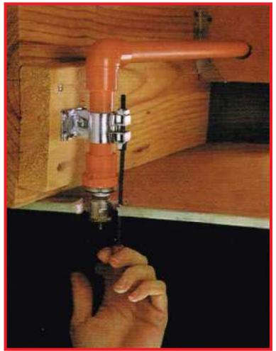
Allows for sprinkler head adjustment after ceilings have been installed.
